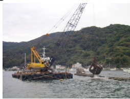
Fig. Work of construction
